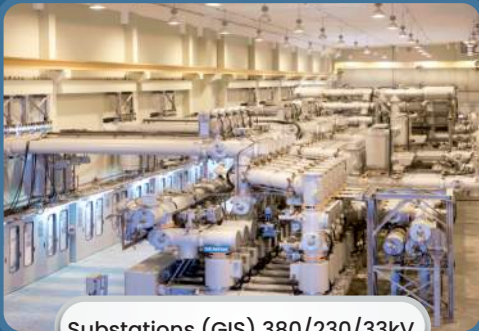
Substations (GIS) 380/230/33kV
